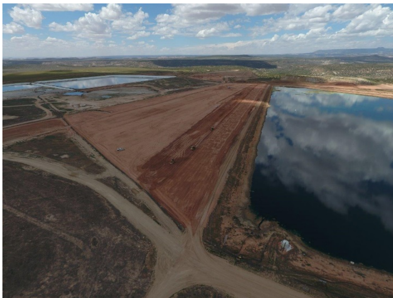
White Mesa Mill Cell 2 Impoundment Reclamation Cover prior to vegetation growth.
