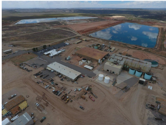
White Mesa Mill near Blanding, Utah (2018)- State of the Art Tailings Cells 4A and 4B in Background; Partially Reclaimed Tailings Cell No.2 between Tailings Cells 4A and 4B and Tailings Cell 1
