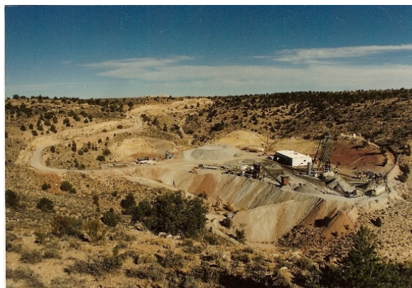
Pigeon Mine Site During Full Production and Ore Sorting November 16, 1989 (view looking north)
