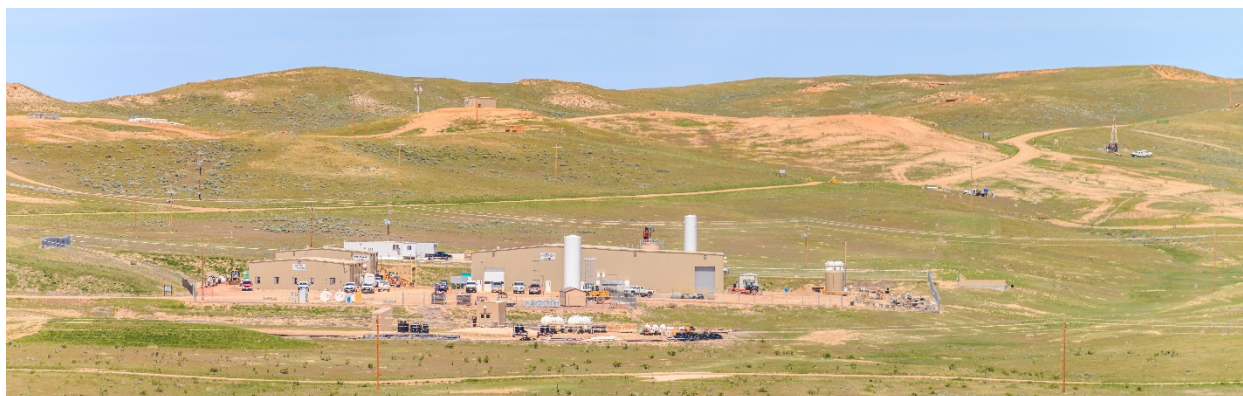
State-of-the-Art Nichols Ranch ISR Project near Linch, Wyoming – approximately 62 miles from Casper, Wyoming
